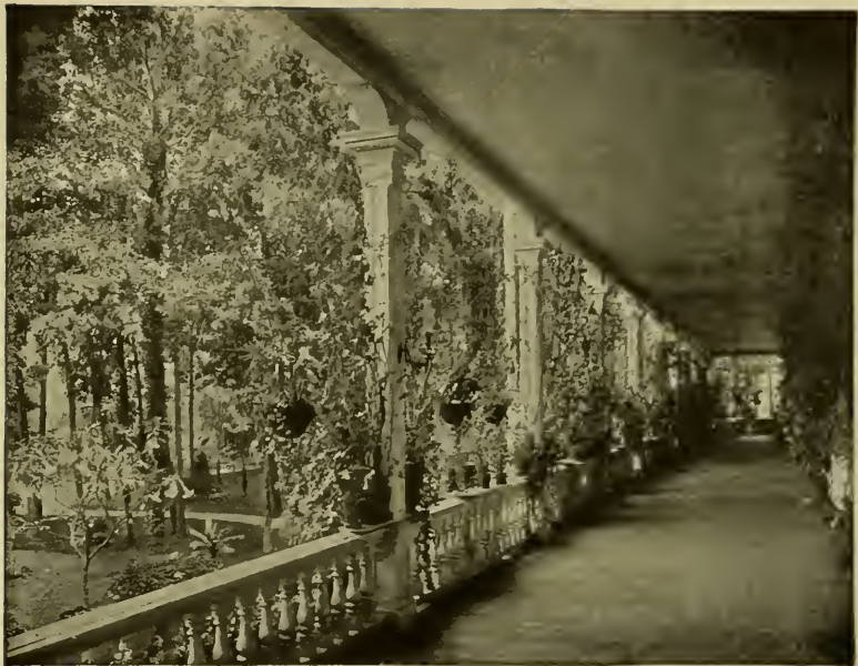
WEST PORTICO, WATER GAP HOUSE, DELAWARE WATER GAP, PA.
